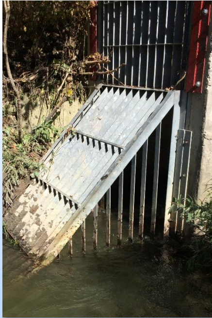
Above left: Trash screen as originally installed. Above right: Newly modified trash screen. The rack is raised, and the new bottom rack (below waterline) has wider spacing between the bars.
